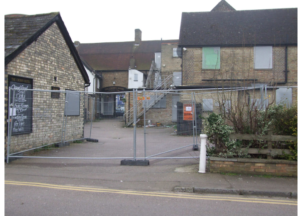
Church Street – fencing across car park entrance
